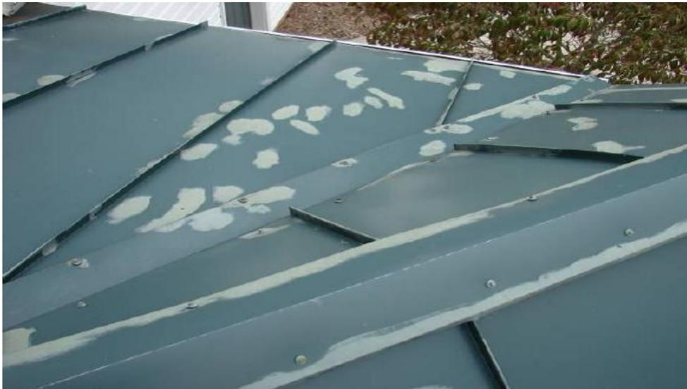
**Figure 1 - Appearance of a pre-coated metal roofing where a low performance field applied air-dry paint system was used**
